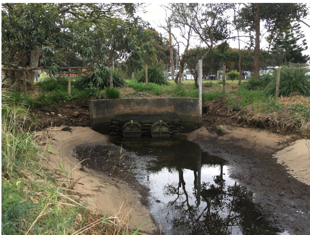
Figure 2.21 Gated Stormwater Outlet at Chainage 970 m
