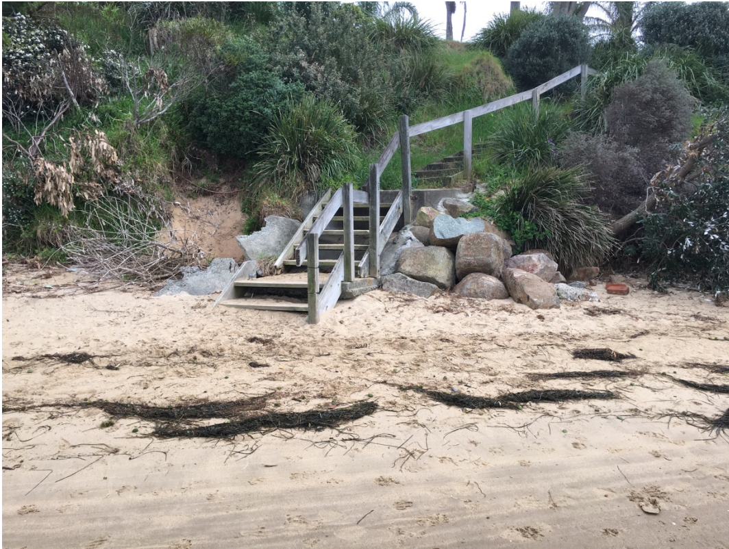
Figure 2.11 Beach Access Opposite Renown Avenue (~Chainage 480 m)
