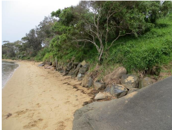
Plate 4: Boulder wall at 64 River Road
