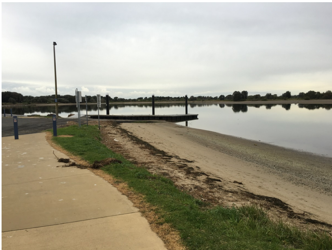
Figure 2.20 Zone 4 Foreshore Profile at Chainage 1000 m, Looking East
