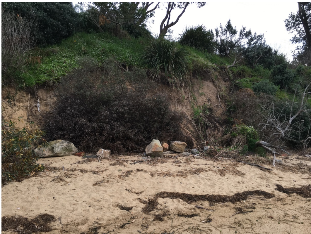
Figure 2.9 Back Beach Embankment in Zone 2B with extensive land-slip (~Chainage 530 m)
