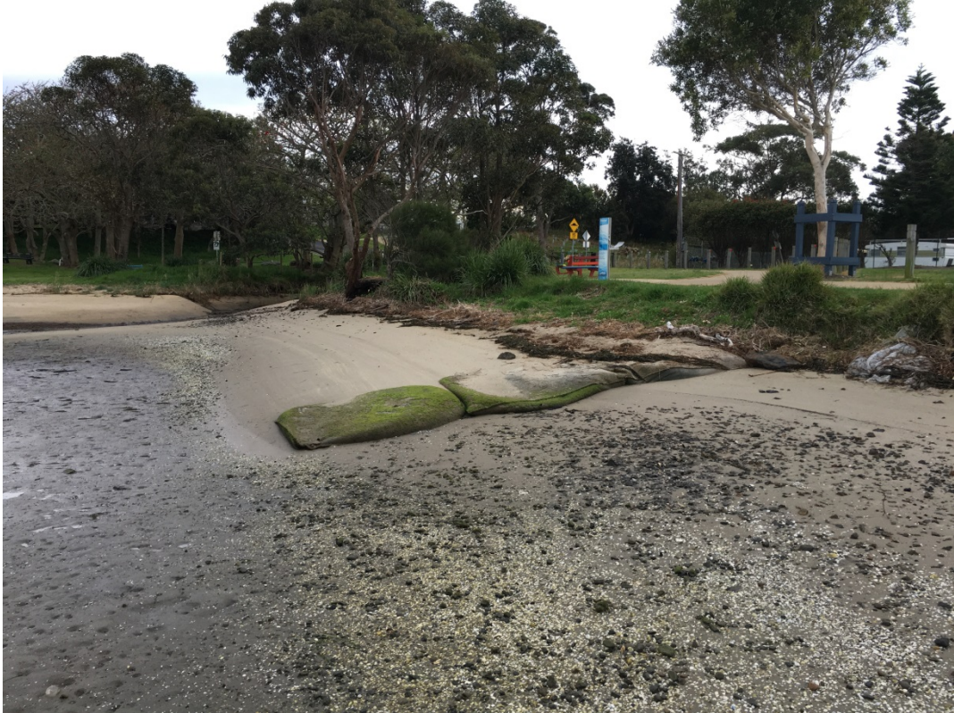
Figure 2.22 Geotextile Bag Groyne at Chainage 990 m
