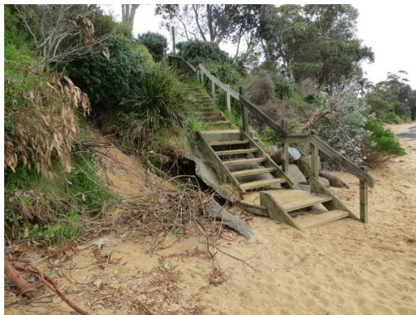
Plate 5: Timber steps (Access 1)
