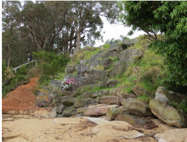
Plate 8: Boulder wall adjacent to Access 2
