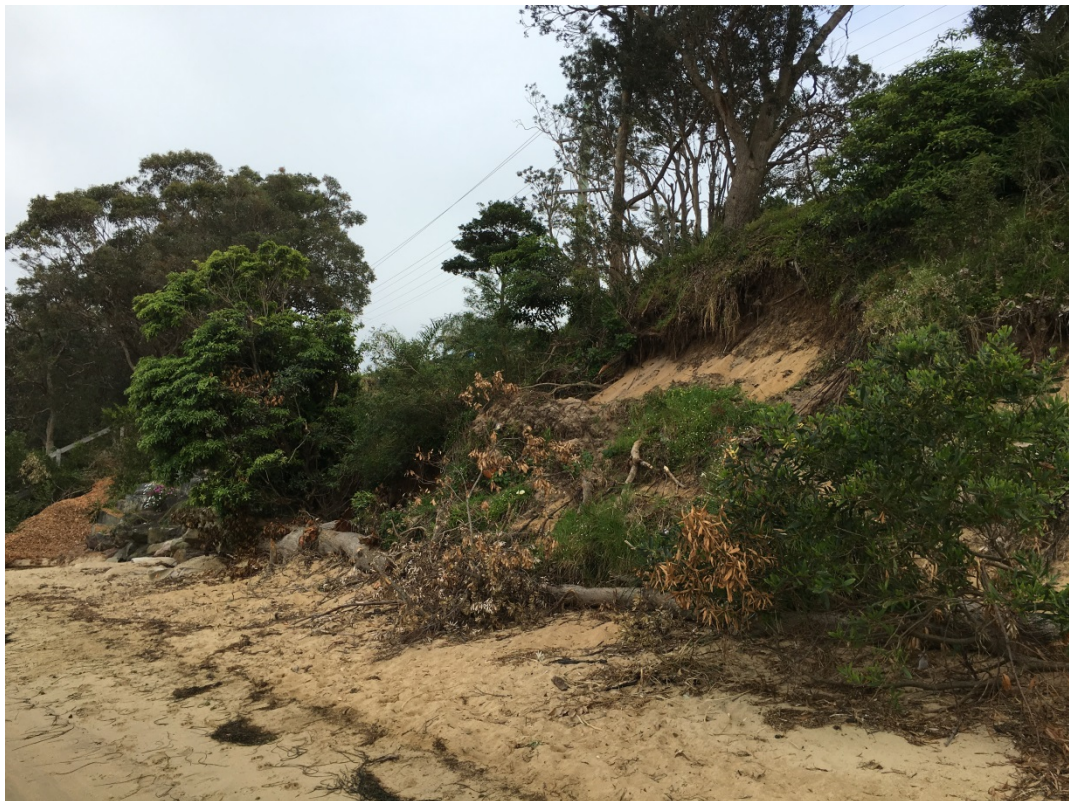
Figure 2.8 Back Beach Embankment in Zone 2B with extensive land-slip (~Chainage 500 m)
