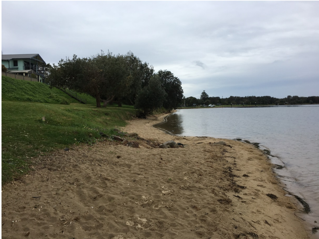
Figure 2.19 Open Stormwater Drain and Rock Rubble at Chainage 810 m
