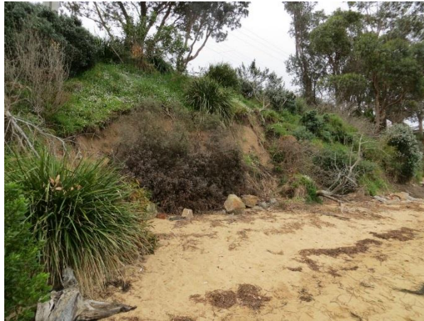
Plate 6: Landslip area north-east of Access 1
